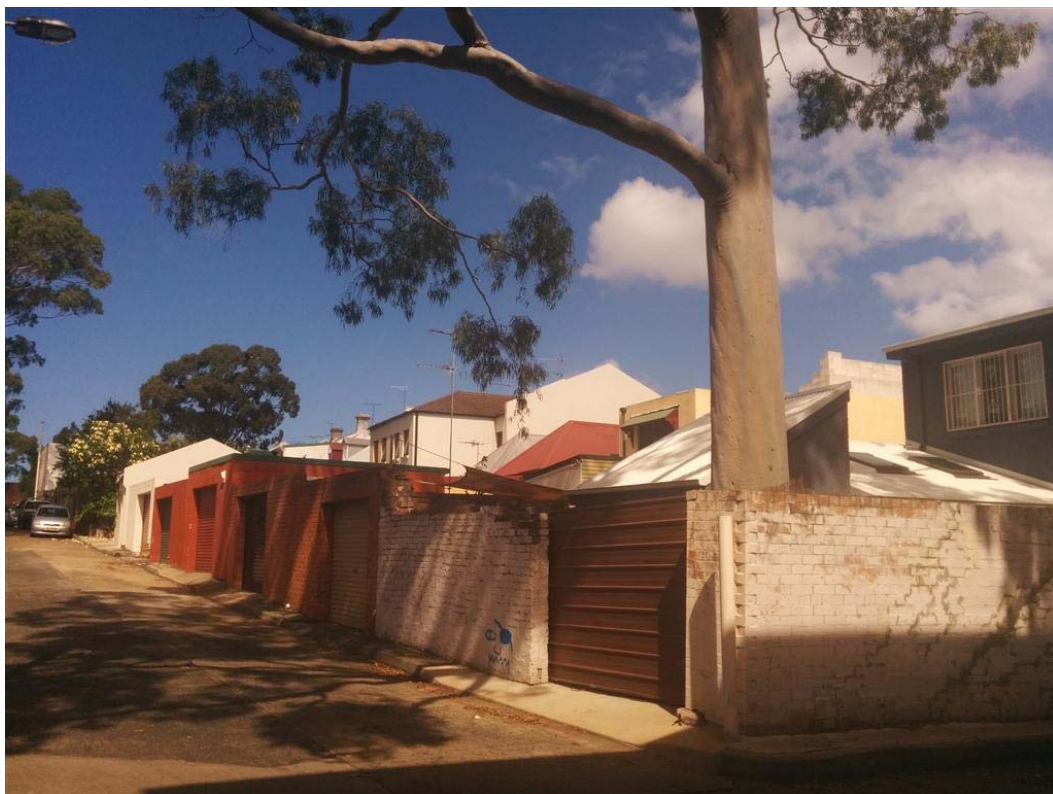
Figure 6: View of Hansard Street terraces from Tosh Lane
