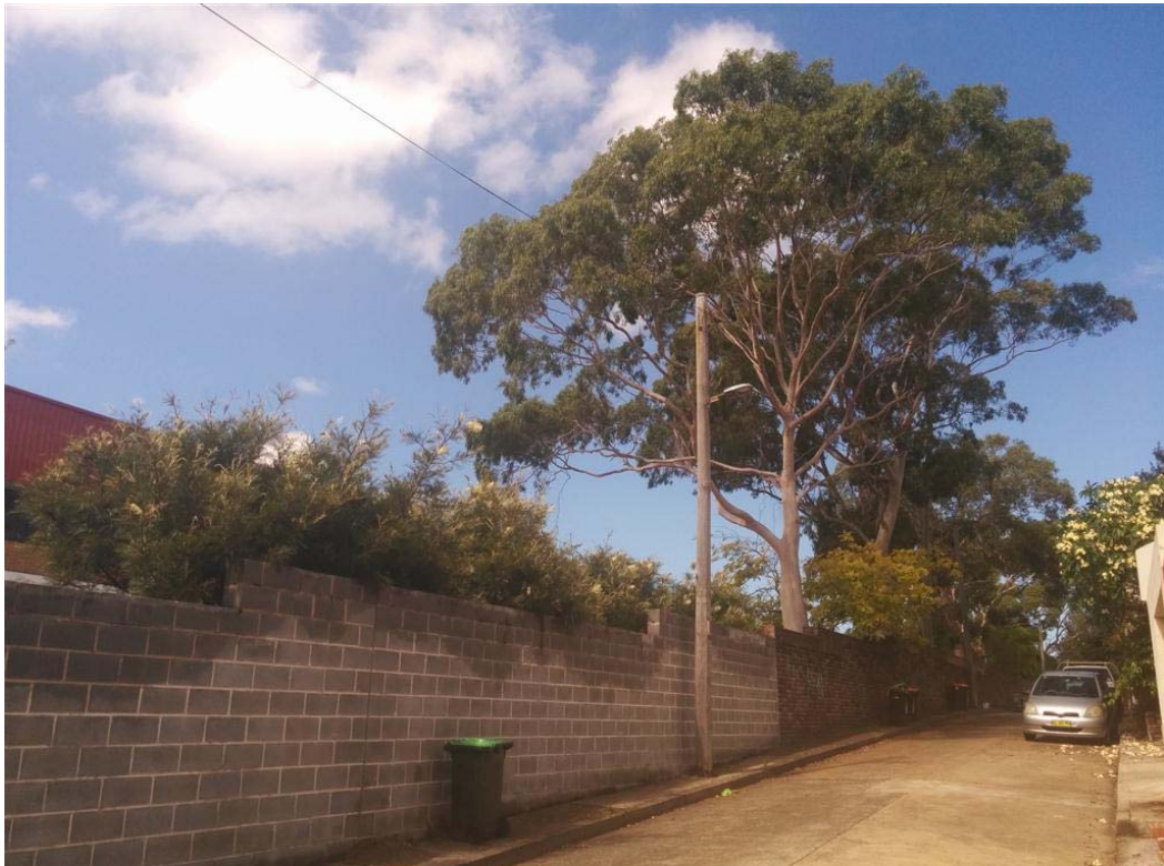
Figure 5: View of existing southern boundary (looking east along Tosh Lane)
