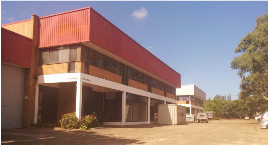
Figure 3: Existing buildings on site
